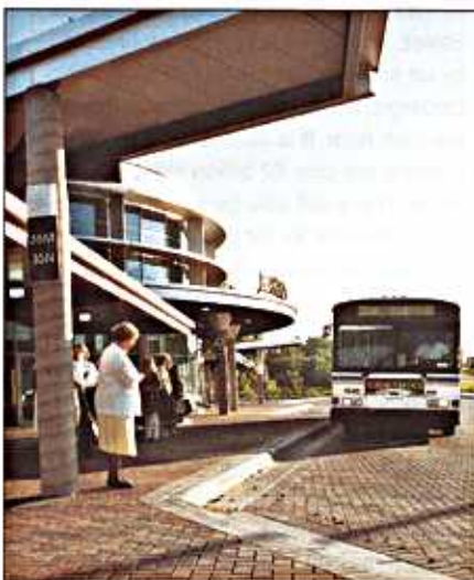
The recently opened Burnsville Transit station (above) interior and exterior
